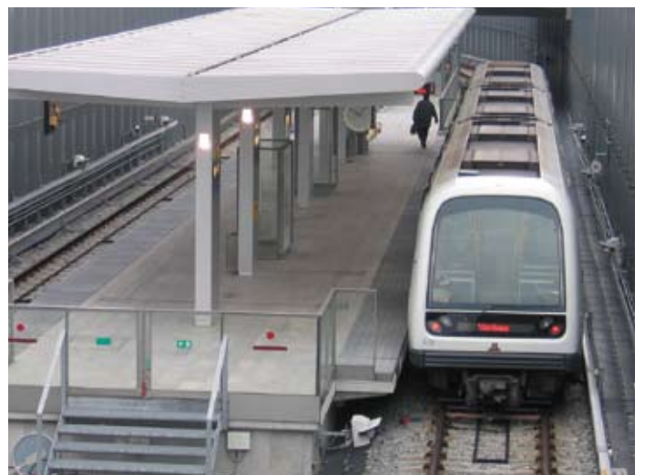
Copenhagen Metro – using RockDelta® anti-vibration mats
